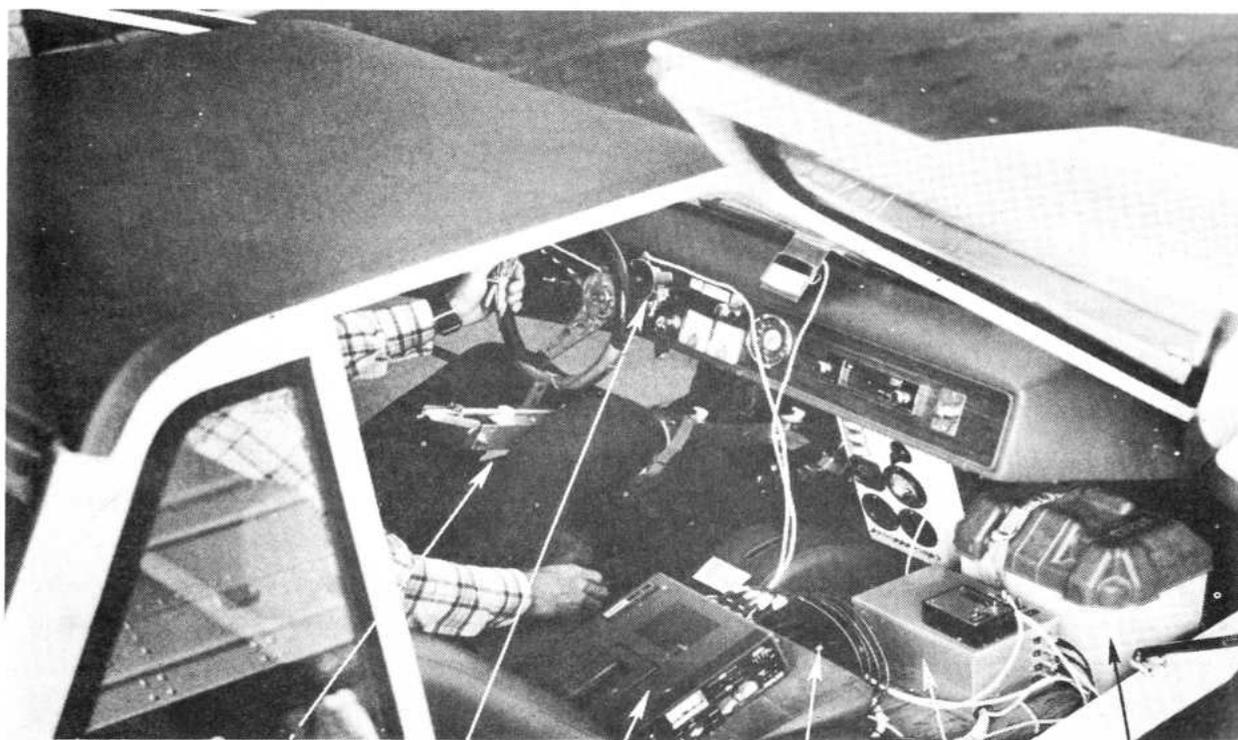
Brake Force Leg      Steering Transducer      Recorder      Inertial Transducers      Calibration Unit      Auxiliary Battery
